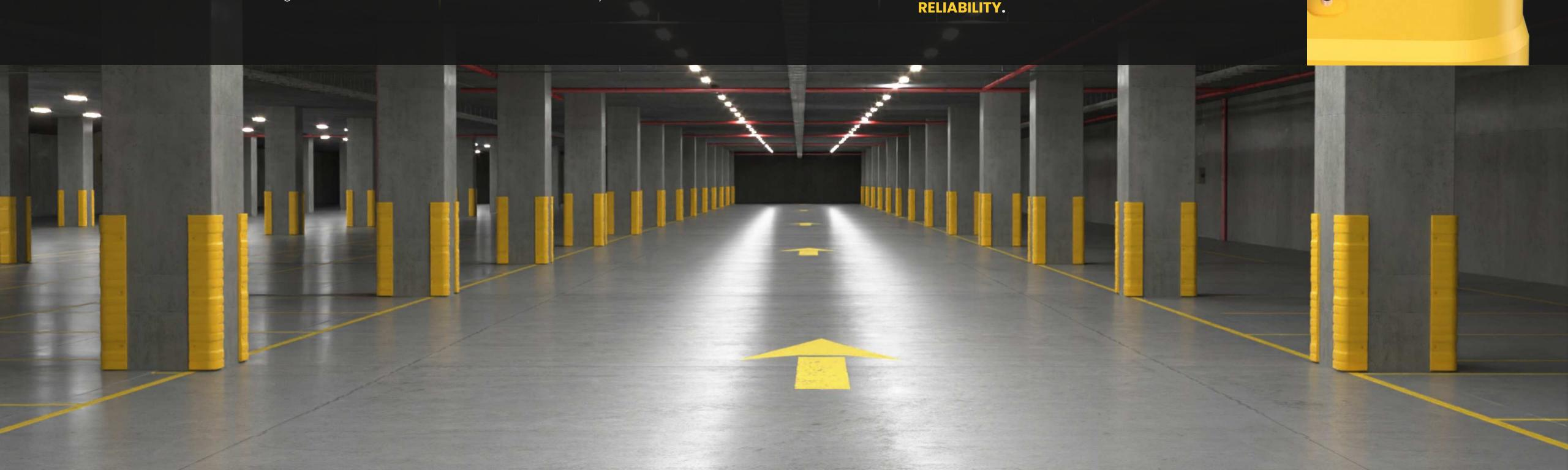
Corner protection barriers are crucial for preventing damage to column edges and reducing costly repairs caused by forklift impacts. They enhance safety, minimize downtime, and improve efficiency by absorbing and dispersing impact forces. Investing in these barriers safeguards structural integrity, protects equipment and personnel, and lowers maintenance expenses, ensuring a safer and more cost-effective work environment.
